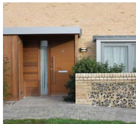
Fig. 58 - Contemporary porch and store cupboard with traditional wall
