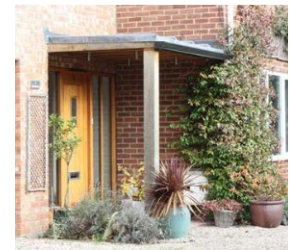
Fig. 59 - Simple modern details concealing the utility boxes
