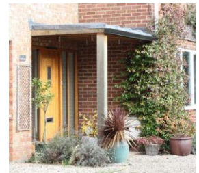
Fig. 59 - Simple modern details concealing the utility boxes
