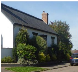
Fig. 52 - Planted street achieved without deep front gardens
